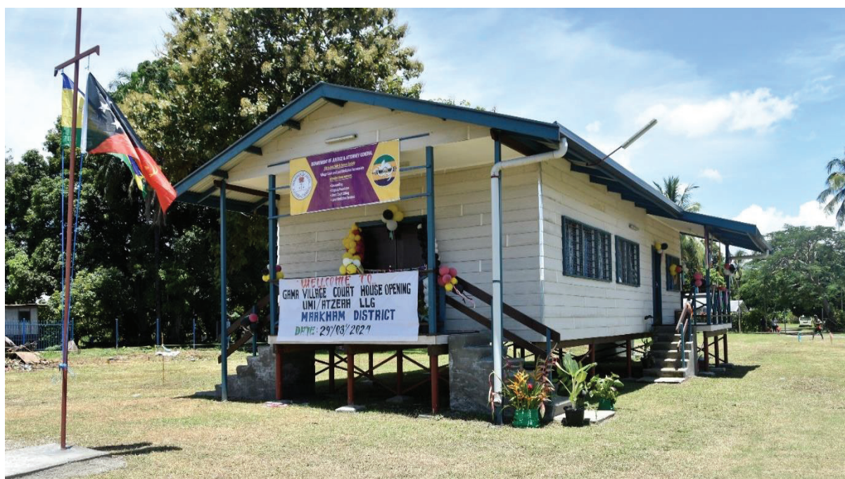
Figure 13: Gama Village Court House, Markham District of Morobe Province built per the Village Courts Policy 2020-2030
